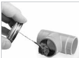
Apply Solvent Cement to Fitting
