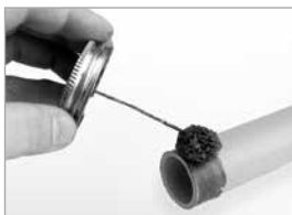
Apply Solvent Cement to Pipe End
